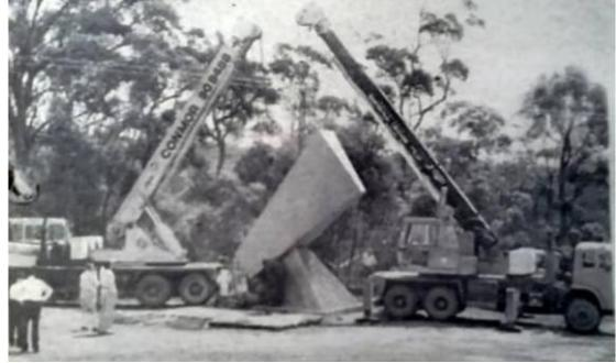
a small mass forming the base, and the larger 21 tonne top section balanced upon it, forming a series of interesting triangles. The two sections were cast on site. Two big mobile cranes inched the massive top section into place, joining precisely on four long retaining bolts locking the massive work together.
